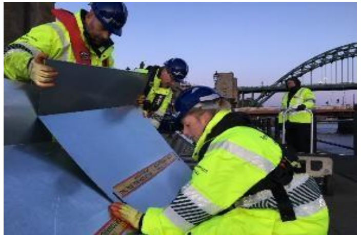
Removable defences being placed on Newcastle Quayside
